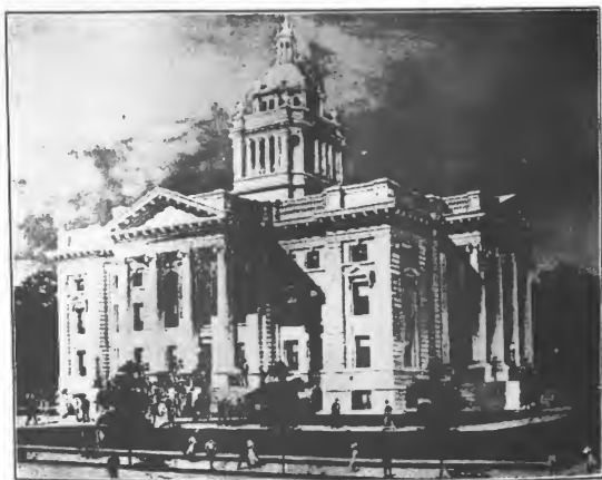
New Court House at Jasper, 1910. (Under Construction, 1909-1910.)
